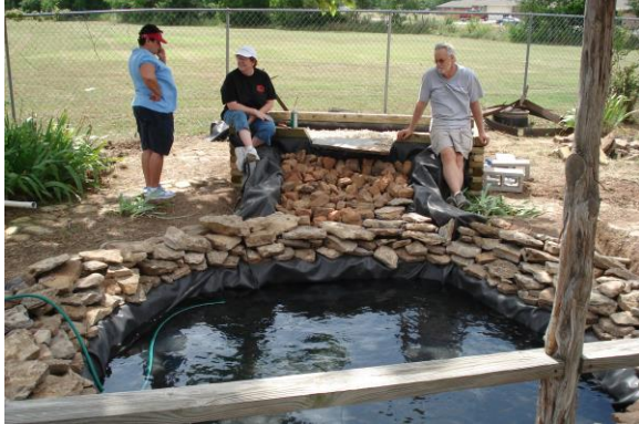
Re-construction is complete and filling with water May 25, 2010.
