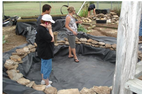
New liner installed and new bog is nearly complete.
