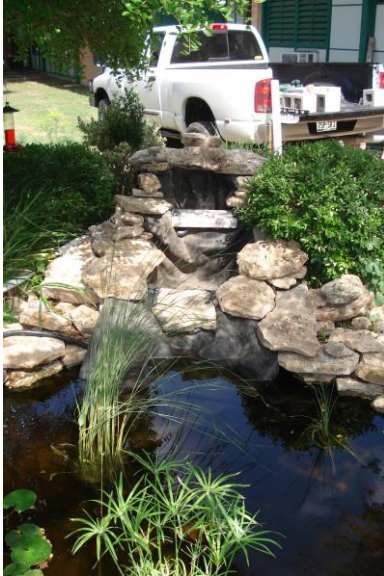
Waterfall under construction
